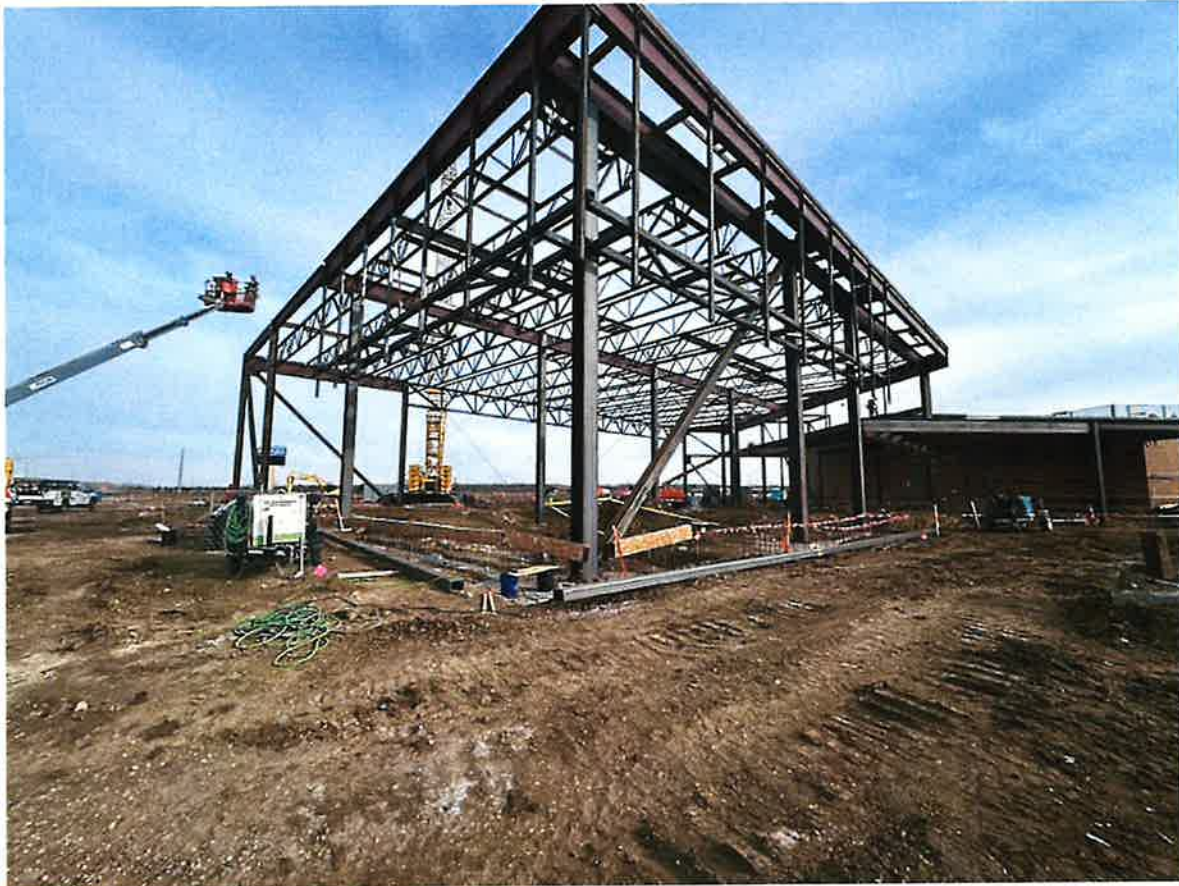
Structural Steel looking south
