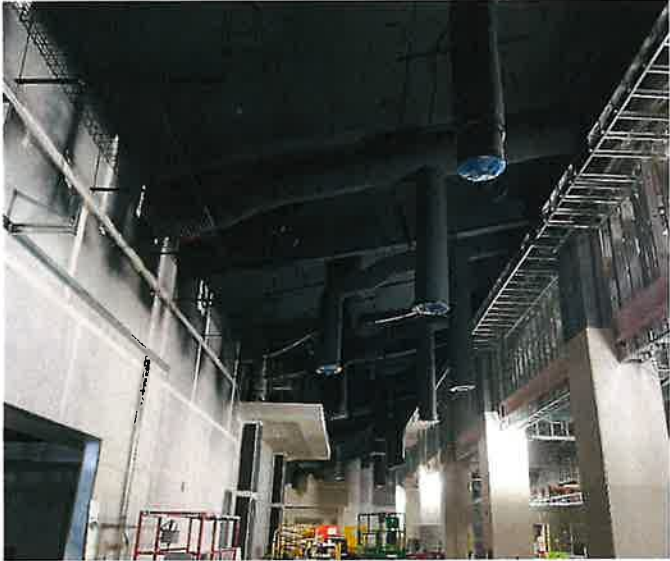
Remodel Exposed Ceiling Black Paint
