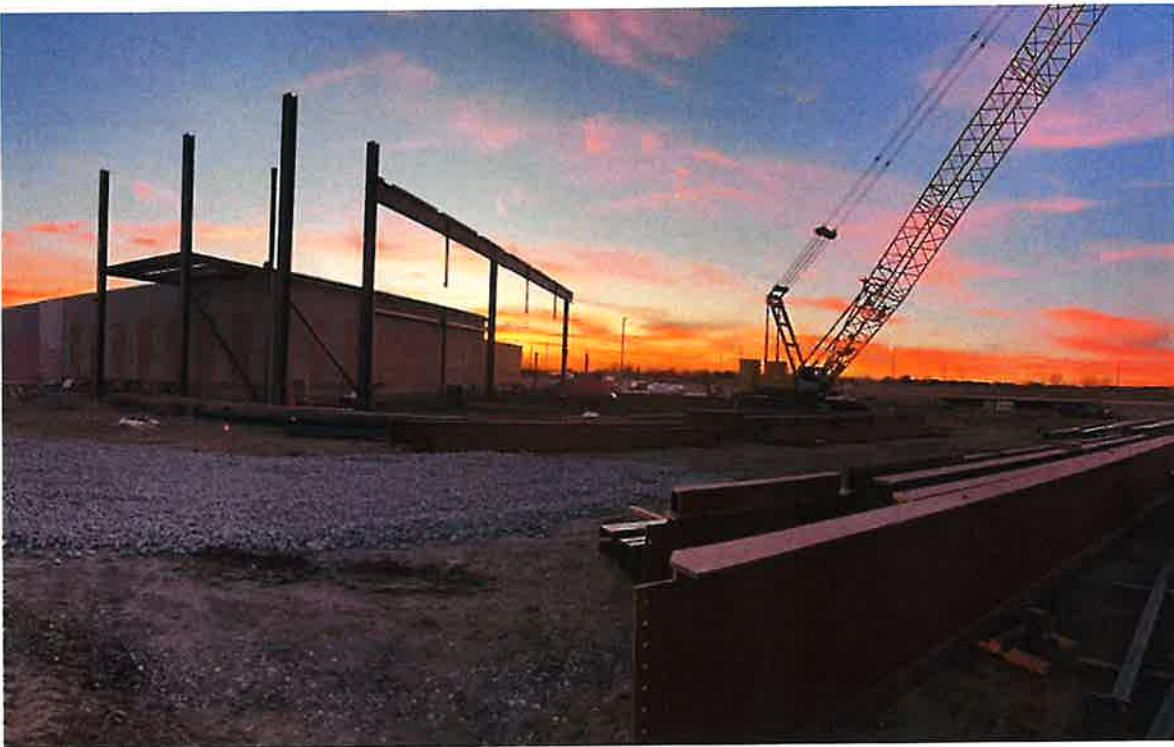
Setting steel on north addition
