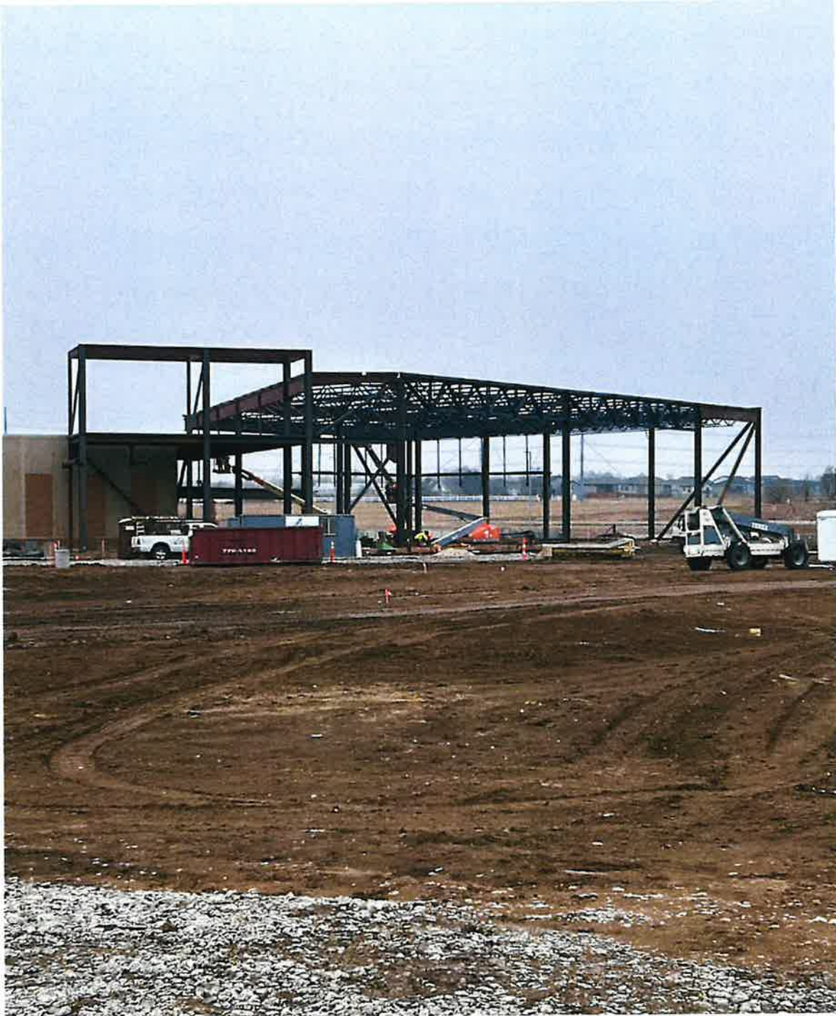
Structural Steel looking West
