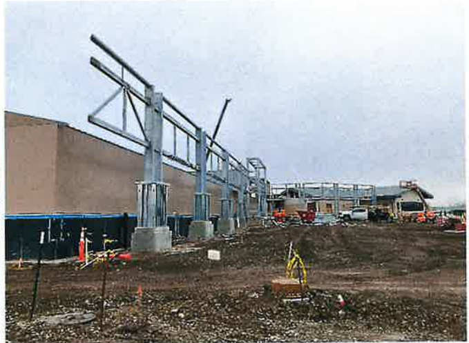
Remodel West Face – Looking South
