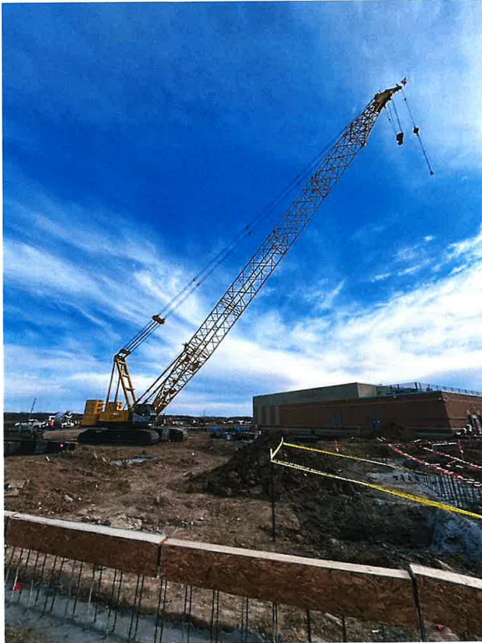
Rebar protection for future stem walls
