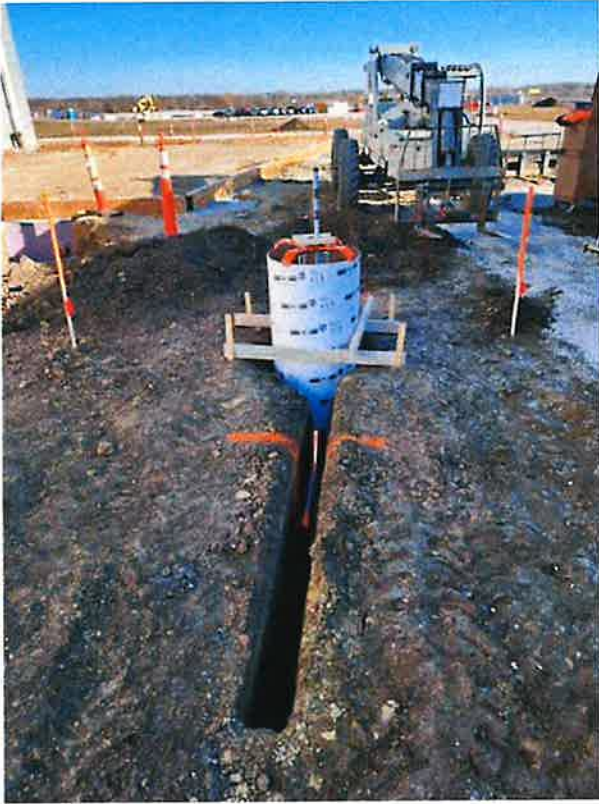
Light pole base at south side of existing building.
