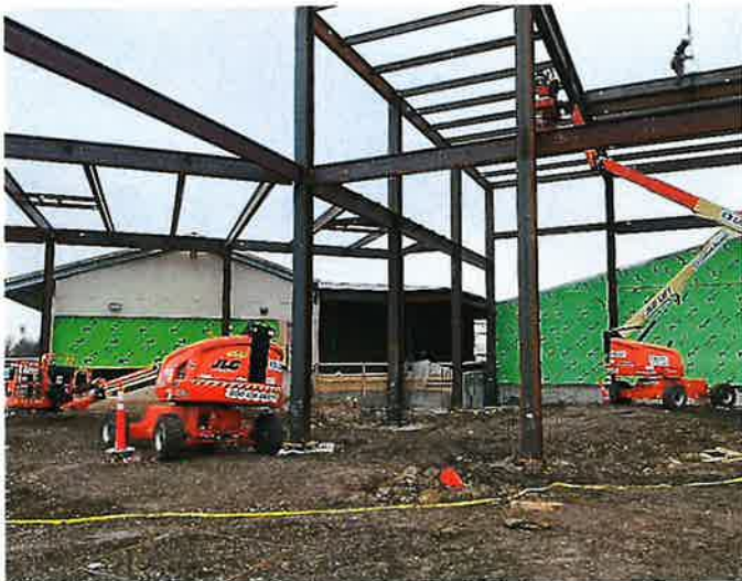
Expansion Structural Steel Erection
