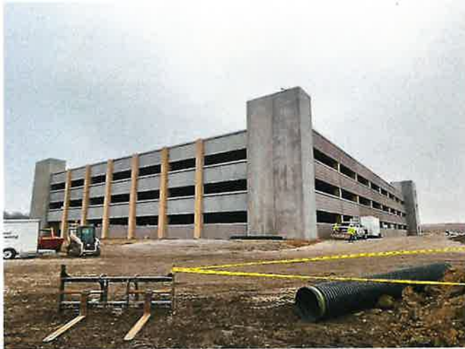
Parking Garage Erection – North/West Face
