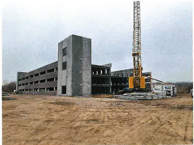
Parking Garage Erection – Interior (Elevator Tower Erected)
