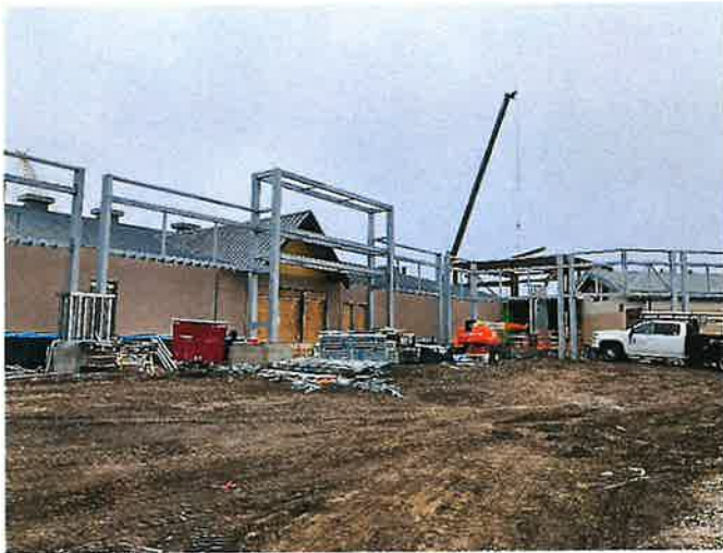
Remodel West Face
