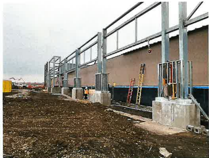
Remodel East Face – Looking South
