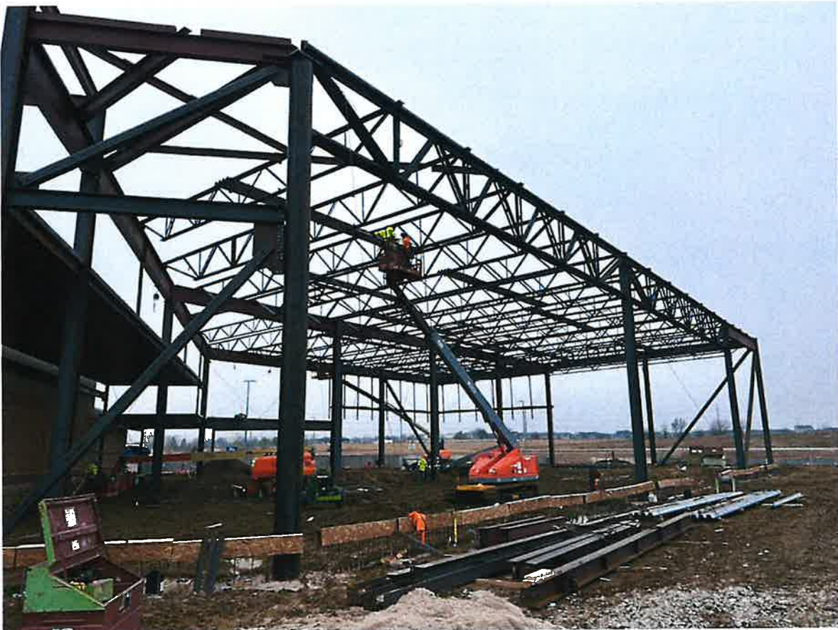
Structural Steel looking West
