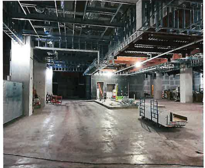
Remodel Main Bar & Gaming Floor Ceiling Framing
