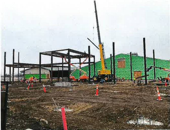
Expansion Structural Steel Erection
