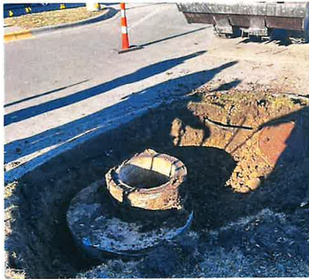
Sanitary sewer on north side of building
